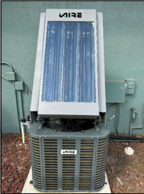
iAIRE model SHRPZ-24LH00A00-A 2-ton condensing unit
